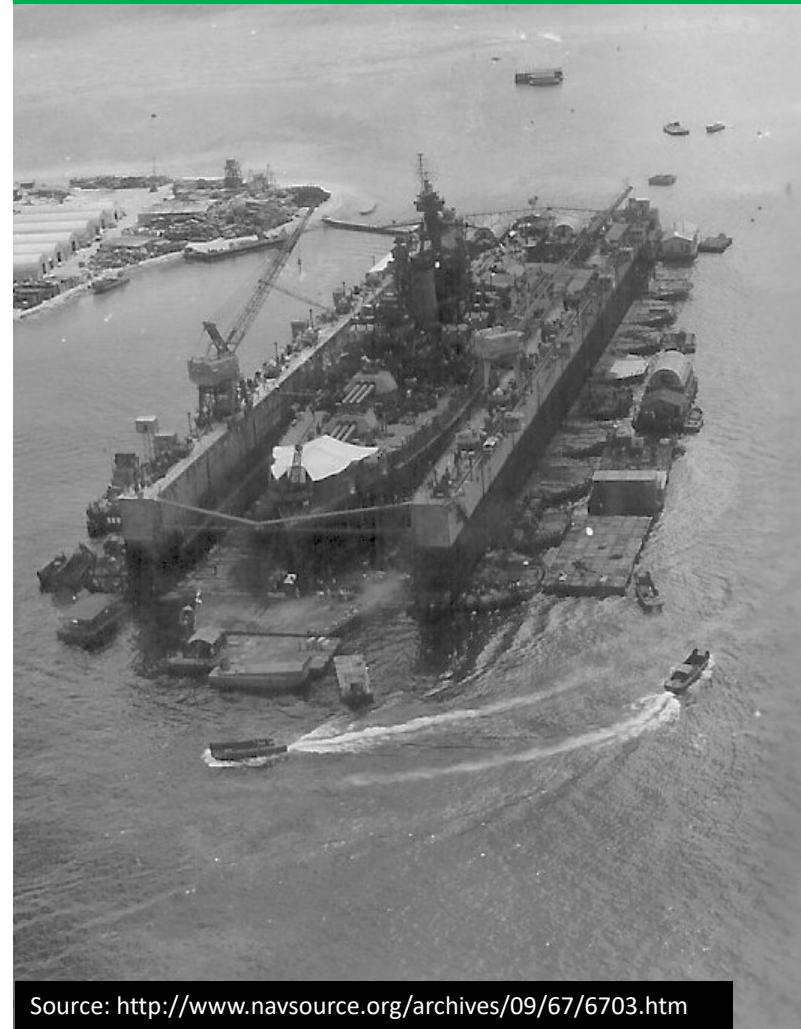
Apra Harbor, Guam (1945): USS ABSD-3 Large Auxiliary Floating Dry Dock repairing USS Pennsylvania after kamikaze attack.
